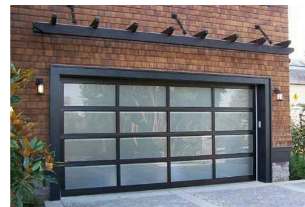
OVERHEAD GARAGE DOOR #10
